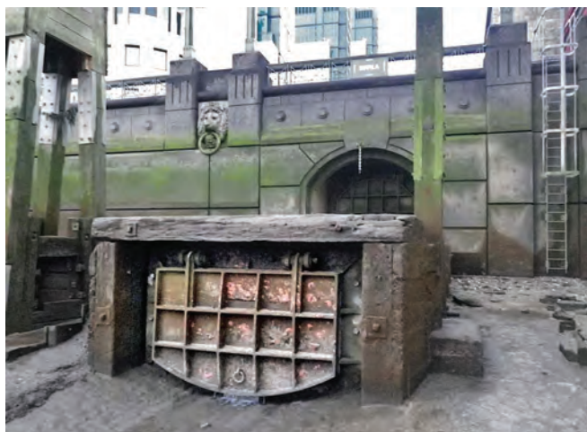
Effra Outfall, Vauxhall Bridge. Photo Bermondsey Bill
